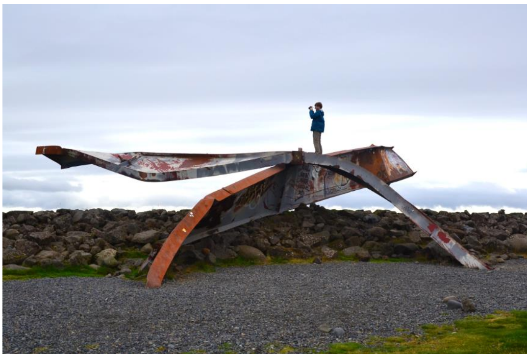
Fig. 4. A fragment of a twisted span of the old bridge that used to cross the Skeiðará river as an evidence of the destructive power of jökulhlaup of 1996, Skeiðarársandur (photo: J. Szafraniec).
